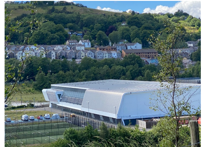
Solar PV Installation at Ebbw Vale Sports Centre
