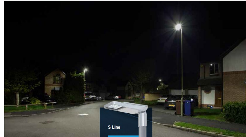
Street Lighting Installation Before and After
